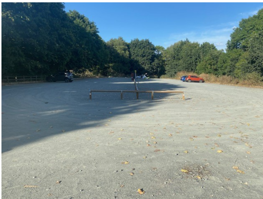
Teston Bridge overflow car park following resurfacing
